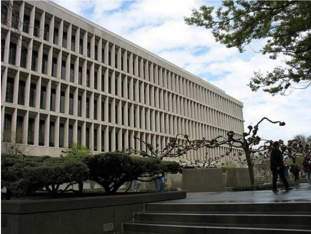
Sacramento County Courthouse
